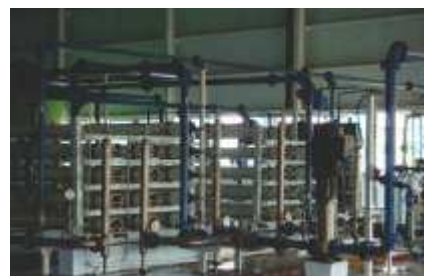
Hyundai Motors - 136.5 m³/hr ETP Recycle along with ZLD Plant
